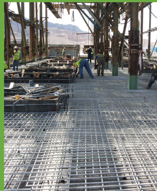
Potash Plant Concrete Slab Replacement, Jordan
